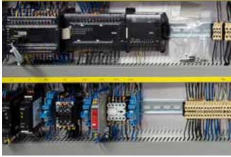
PLC controlled operations functions and monitoring of the unit. Standardised modules and worldwide electrical configurations.
